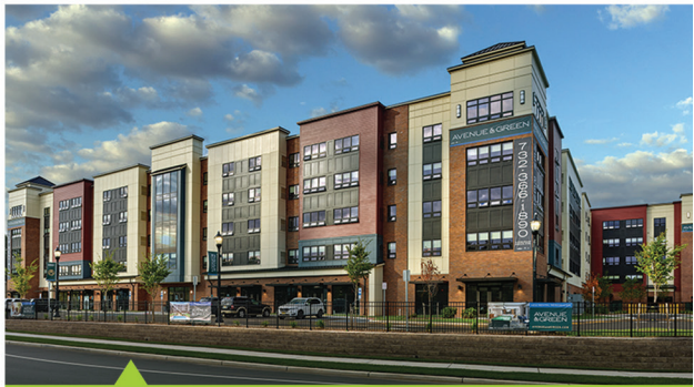
AVENUE & GREEN | WOODBRIDGE, NJ
